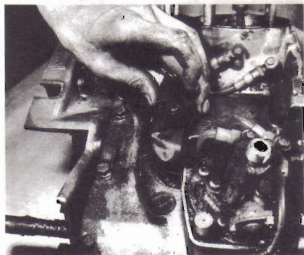
30.3. A metal cover protects the main run of the individual oil pipes
